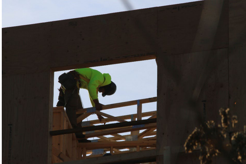
Photo 5. Worker in a frame
